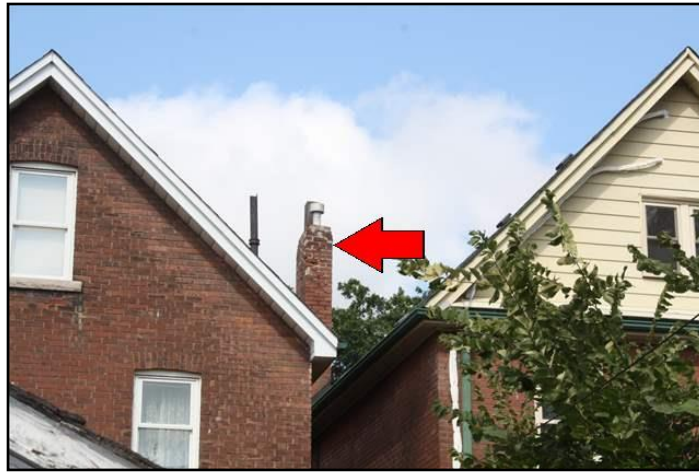
25. Loose, missing or deteriorated masonry
