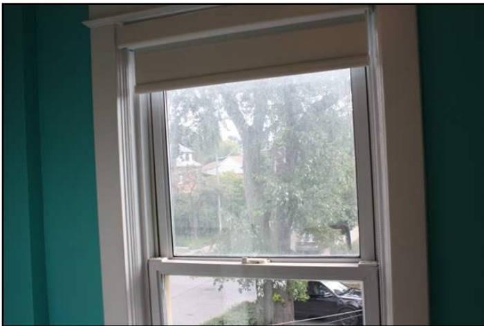
33. Lost seal on double or triple glazing
