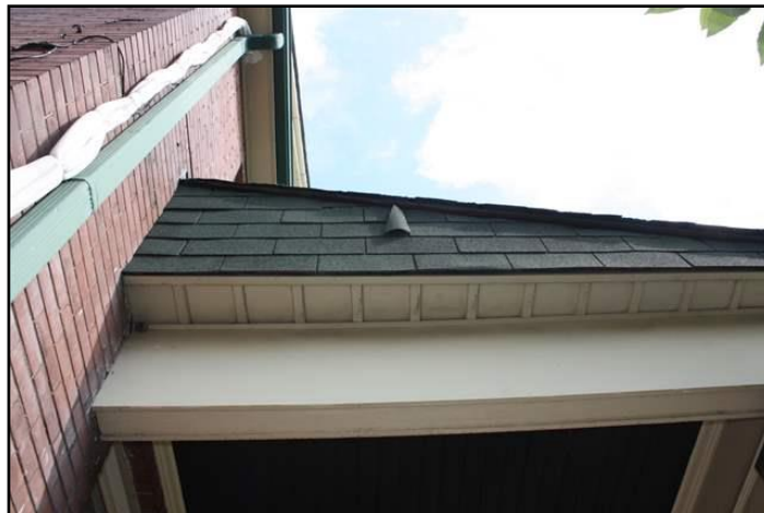
10. Loose, missing or torn tabs
