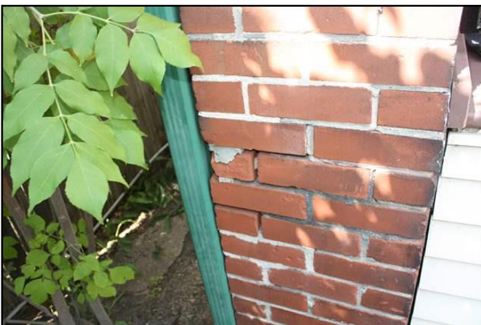
19. Masonry deteriorated
