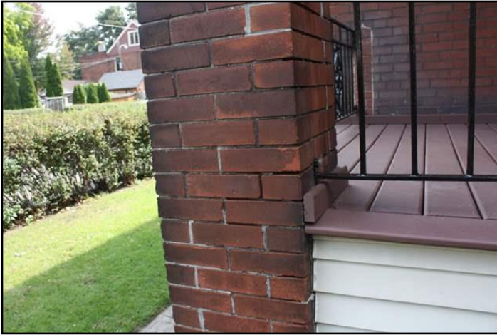
8. Mortar deterioration
