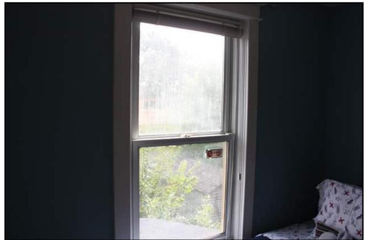
34. Lost seal on double or triple glazing
