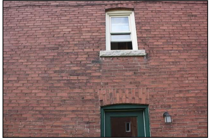
9. Mortar deterioration
