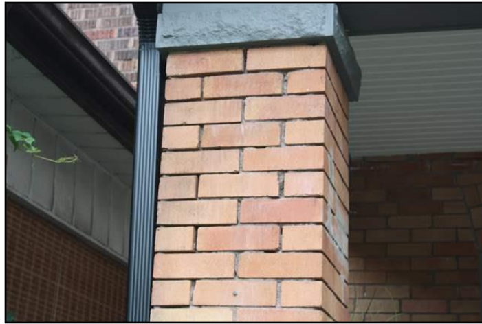
1. Mortar deterioration
