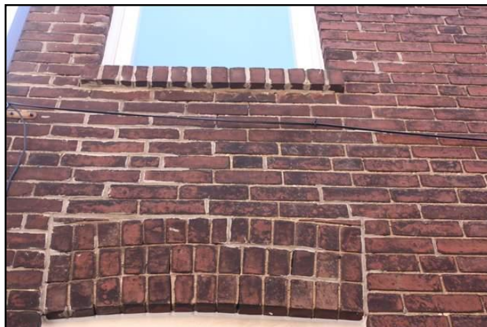
5. Mortar deteriorated
