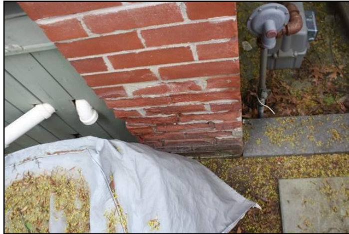
5. Spalling
