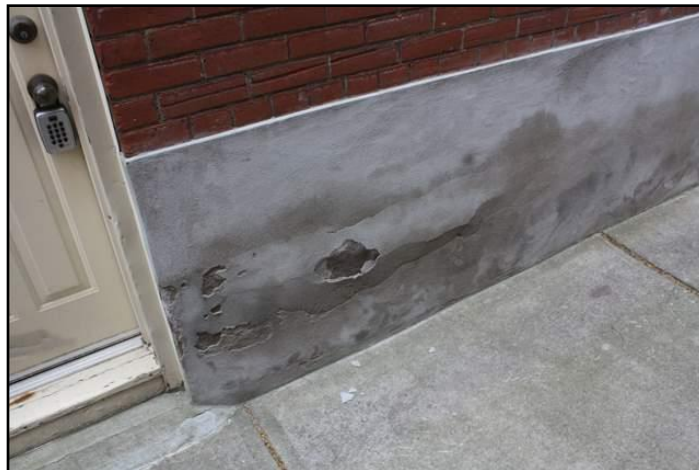
7. Parging damaged or missing
