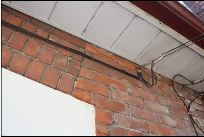
7. Spalling
