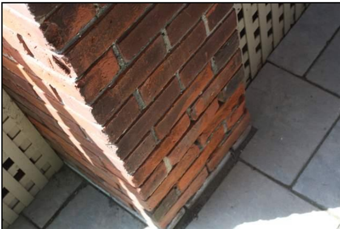
5. Spalling
