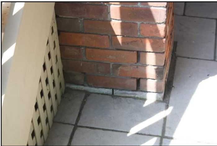
9. Missing mortar
