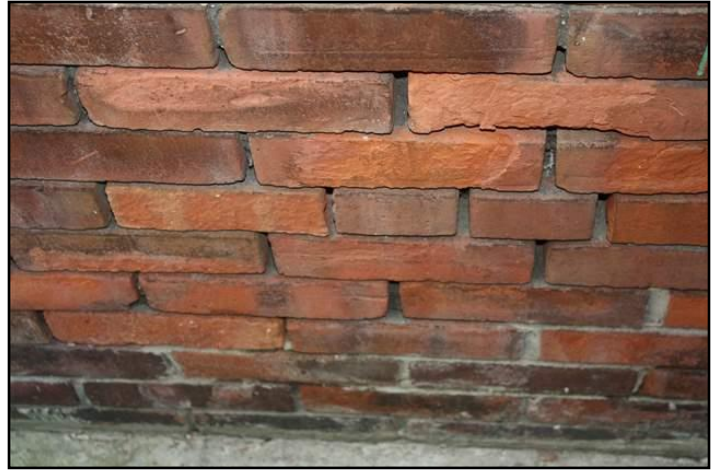
8. Spalling
