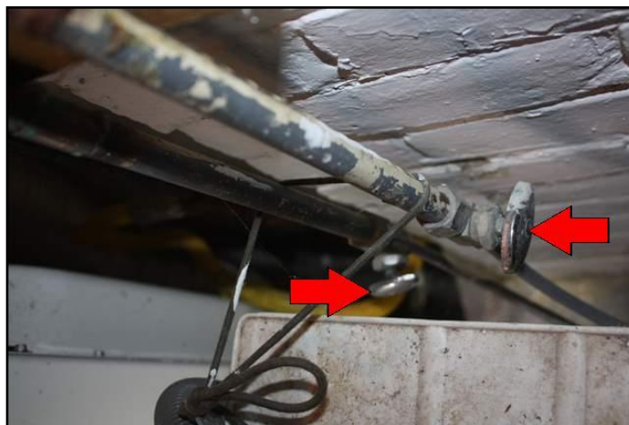
18. isolation valves are off
