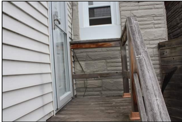
12. Spindles (balusters) climbable
