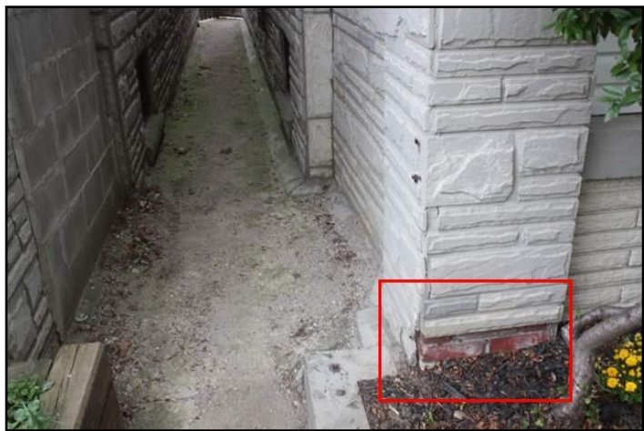
7. Spalling
