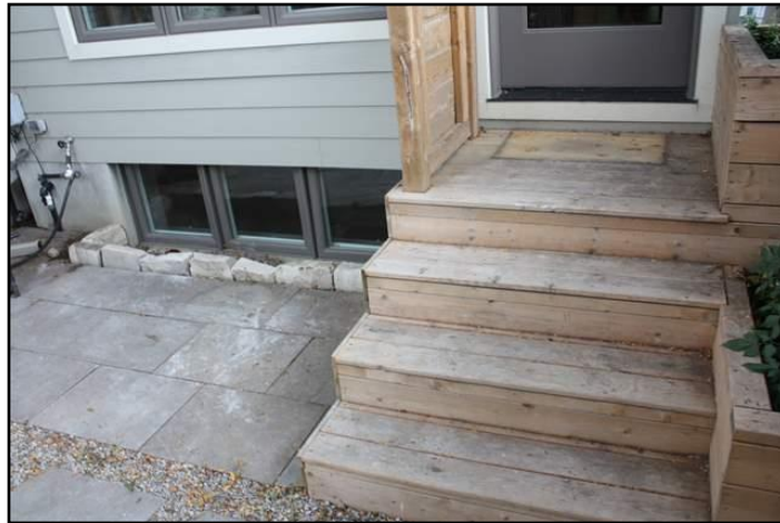
3. Missing Handrail
