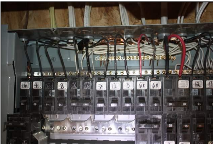
11. No links for multi-wire circuits
