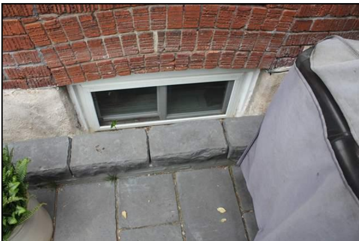
6. Sill - Near or at Grade Level
