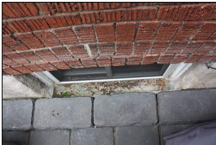
7. Sill - Near or at Grade Level
