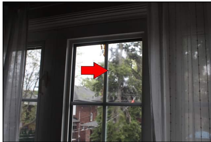
22. Lost seal on double or triple glazing
