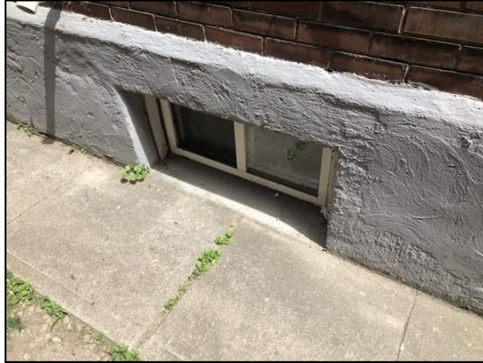
13. Sill - Near or at Grade Level
