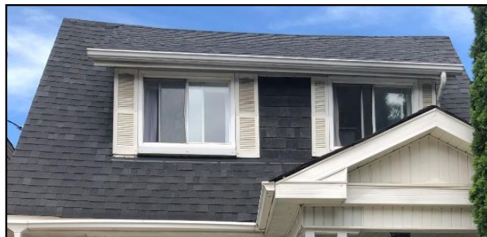
2. Asphalt shingles 5 years old
