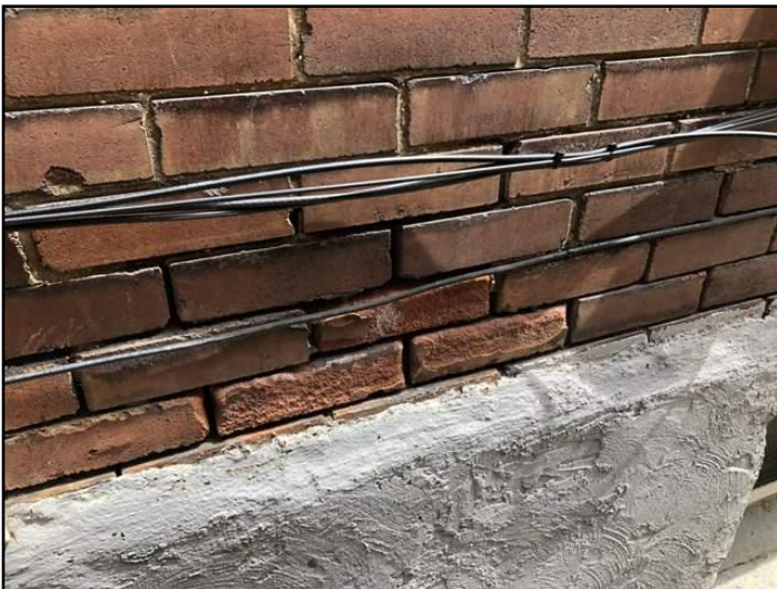
11. Spalling example
