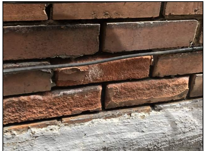
12. Spalling example
