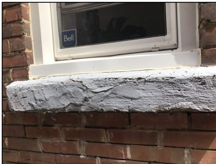
16. Sill deteriorated
