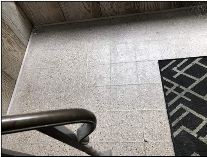
32. Possible asbestos containing materials
