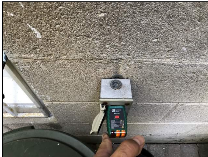
17. GFCI/GFI needed (Ground Fault Circuit...
