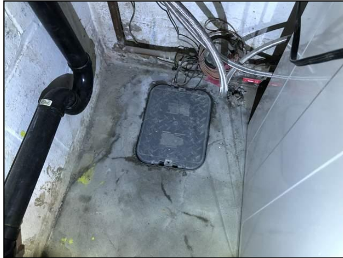
23. Present. These valves help prevent sewer...
