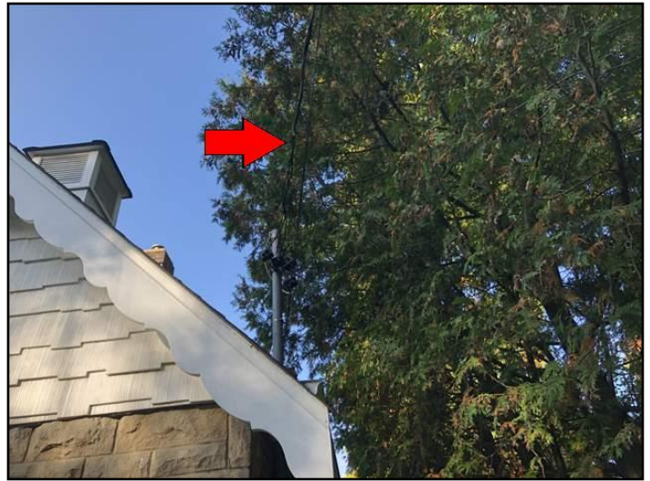
12. Branches / vines interfering with wires
