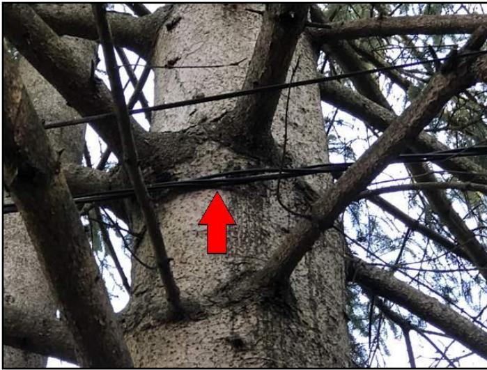
11. Branches / vines interfering with wires
