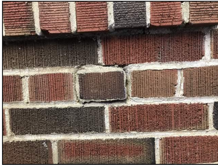
3. Mortar deterioration
