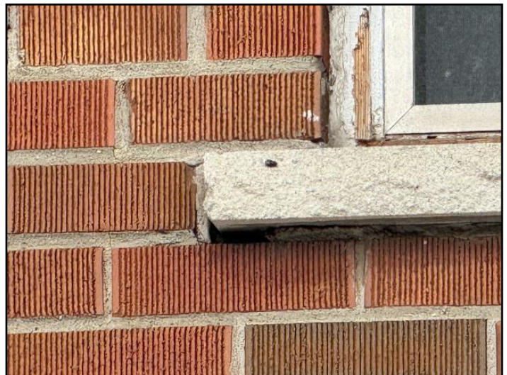
13. Masonry and/or mortar deterioration
