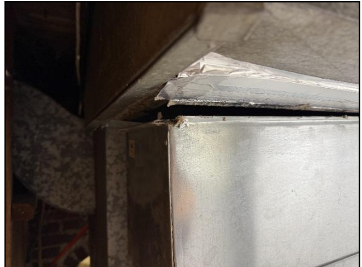
49. Disconnected ducts
