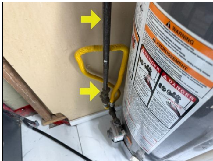
54. Inadequate support
