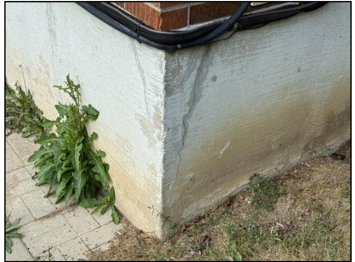
30. Typical Wedge Cracks
