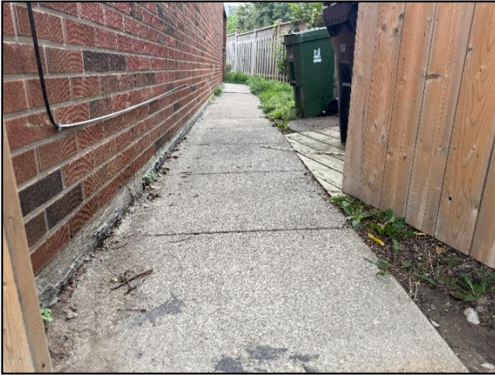
19. Improper slope or drainage
