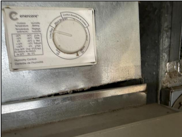
48. Disconnected ducts
