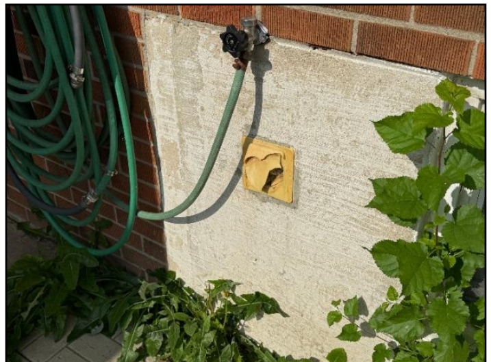
25. damaged vent
