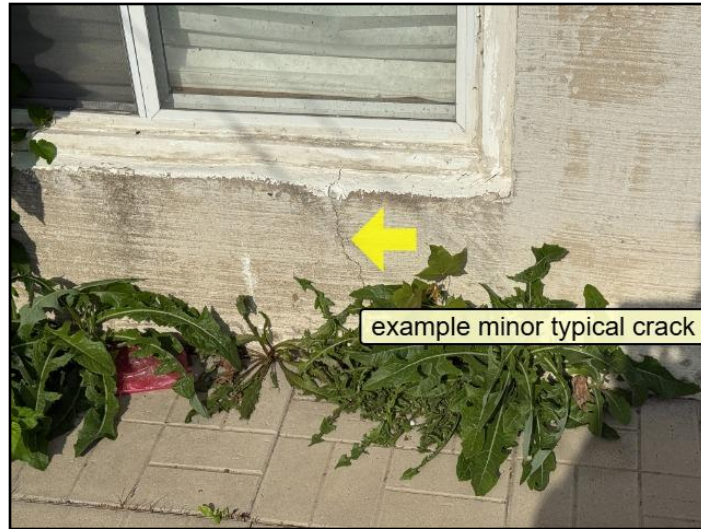
28. Typical minor cracks example
