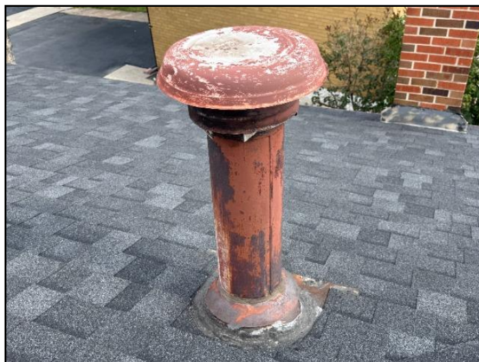
51. Chimney walls rusting and treated with...
