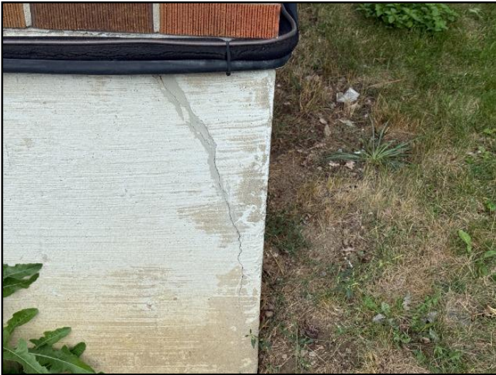
29. Typical Wedge Cracks
