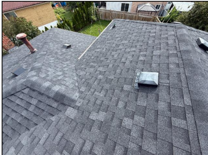
2. Asphalt shingles -- Good condition
