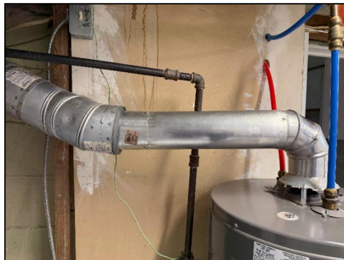
56. Poor slope
