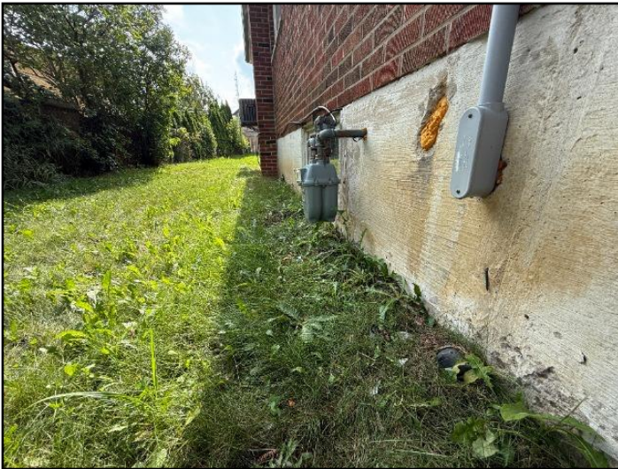
17. Improper slope or drainage
