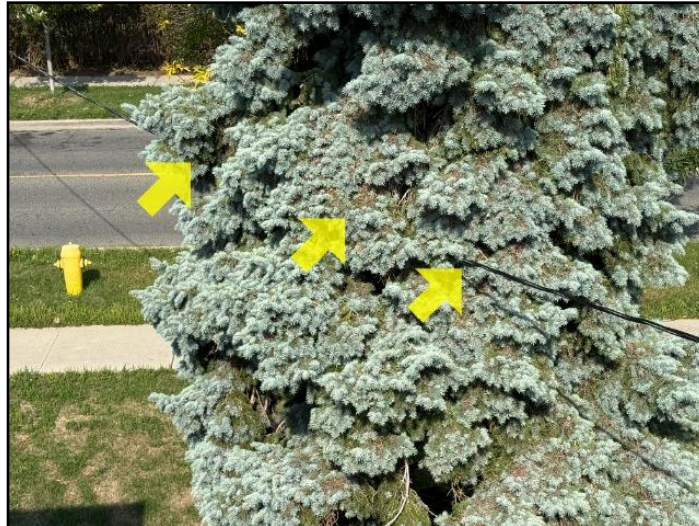
39. Branches / vines interfering with wires
