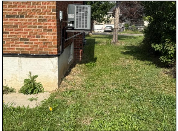
18. Improper slope or drainage
