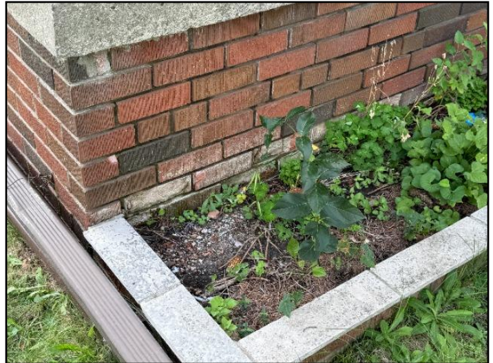
11. Masonry and/or mortar deterioration
