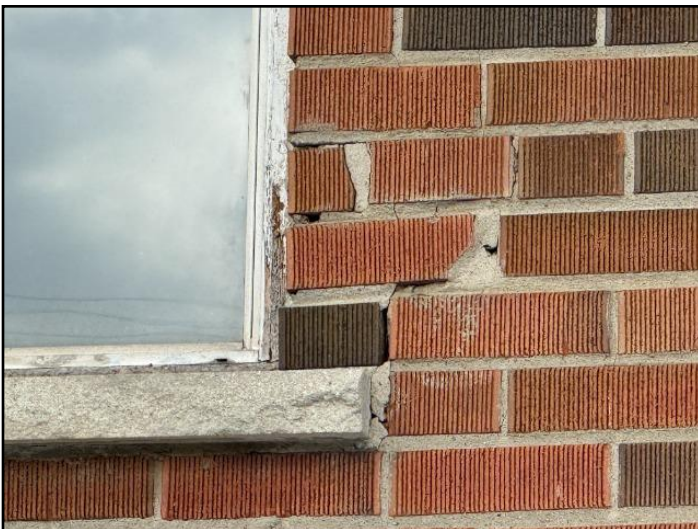
12. Masonry and/or mortar deterioration
