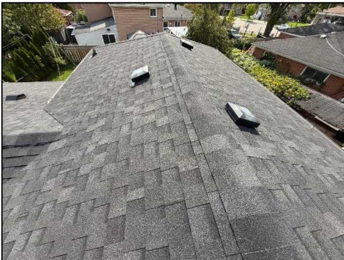
3. Asphalt shingles -- Good condition
