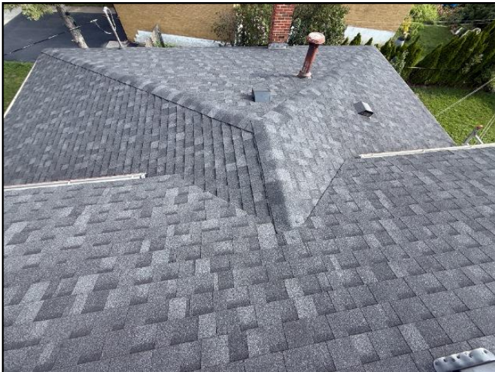
1. Asphalt shingles -- Good condition
