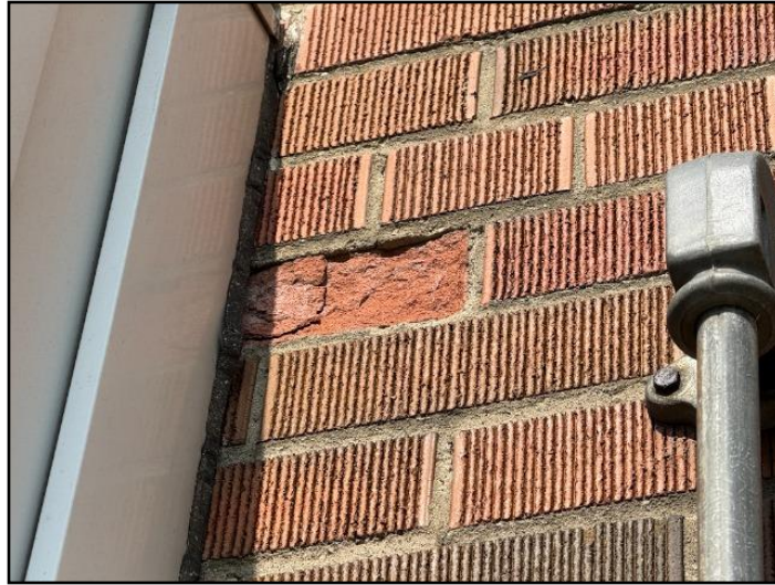
14. Masonry and/or mortar deterioration
