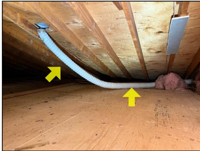
62. Not insulated in unconditioned space
