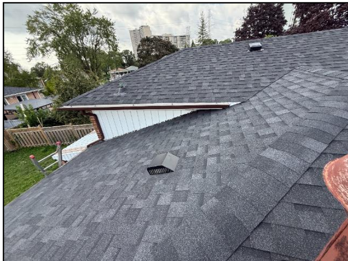
4. Asphalt shingles -- Good condition
