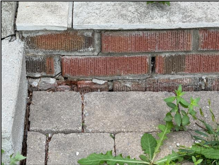
10. Masonry and/or mortar deterioration
