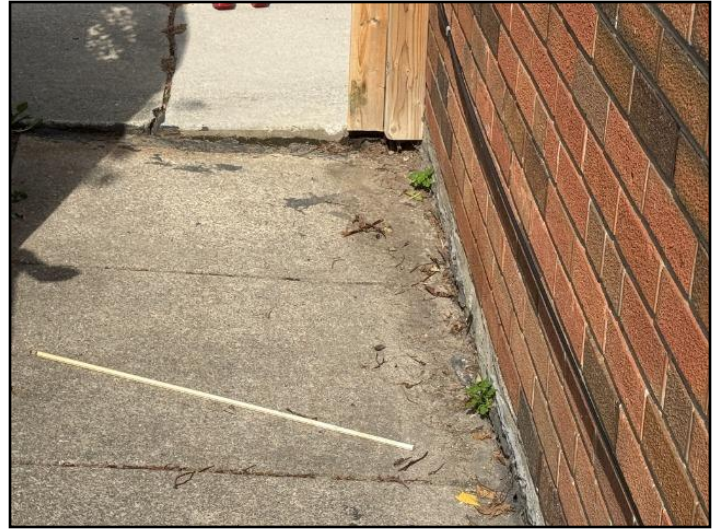
20. Improper slope or drainage
