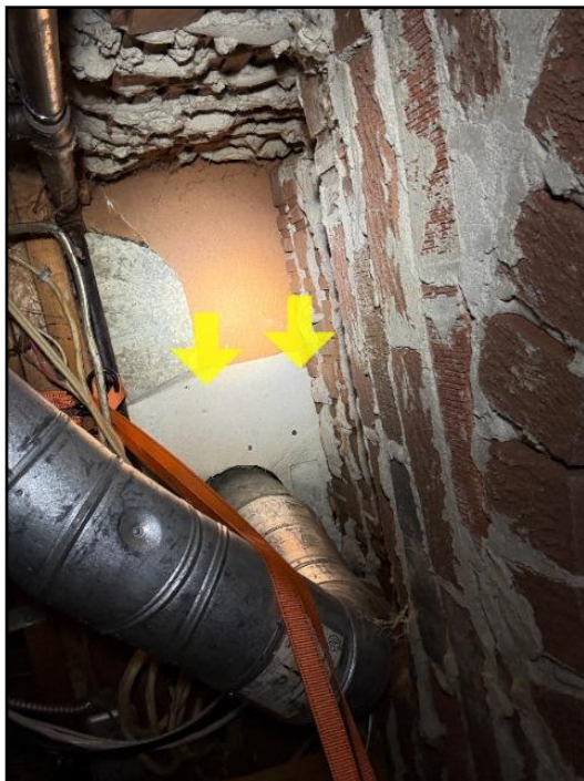
64. Possible asbestos containing materials
