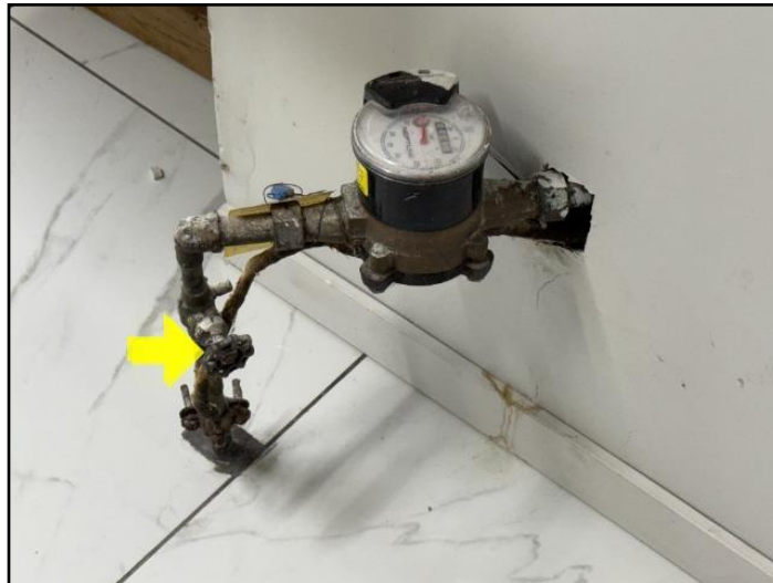
53. Main water shut off valve - Basement
