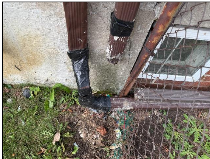
8. Should discharge 6 feet from building
