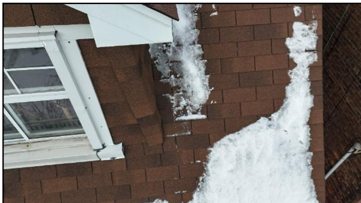
12. Snow on the Roof
