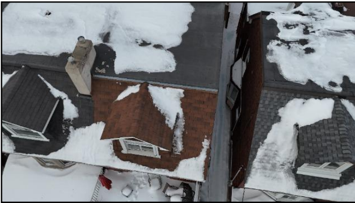
1. Asphalt shingles
