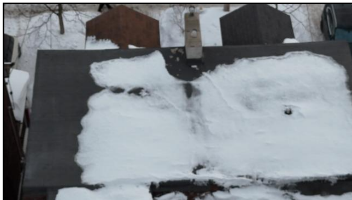
9. Snow on the Roof
