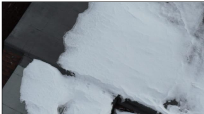
13. Snow on the Roof
