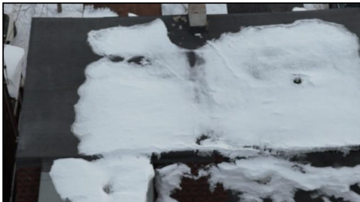
10. Snow on the Roof
