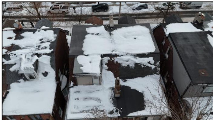
11. Snow on the Roof
