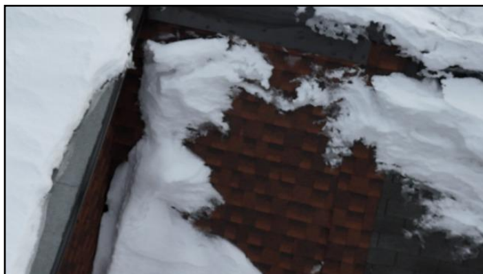
14. Snow on the Roof
