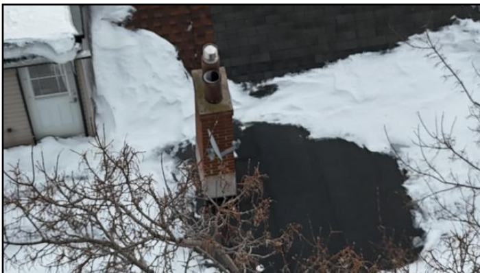
8. Snow on the Roof
